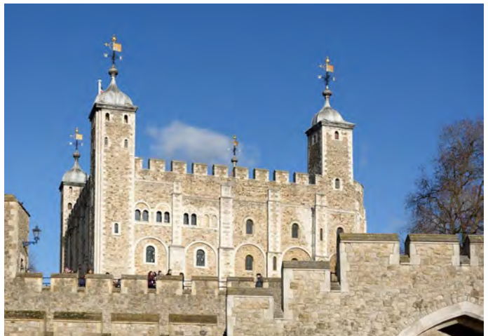
Tower of London: The White Tower with quins, window surrounds etc of dressed Caen stone from Normandy (Jurassic) with Kentish ragstone rubble infill.
