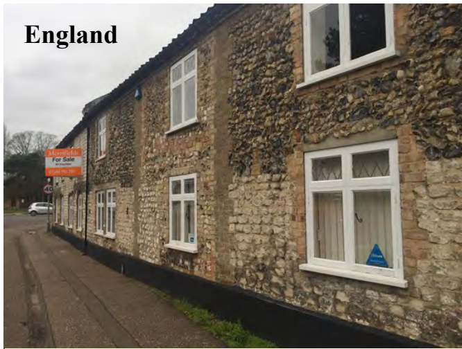
Chalk and flint construction in Thetford, Norfolk, England
