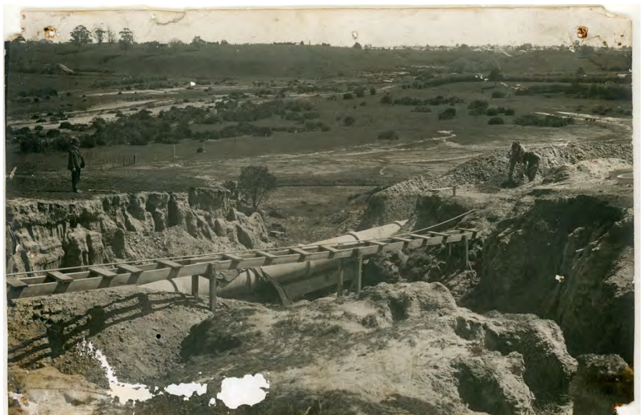
Note sludge in distant Yarrowee Creek, Ballarat. Also showing one of the extensive water races bringing water for puddling (as the miners appear to be doing) and the pipe for drainage of waste water. Also note the erosion and lack of vegetation.
